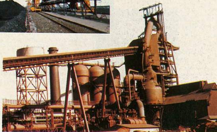
No. 5 BLAST FURNACE AIS Port Kembla ( Inner volume 2,656 m 3 )
