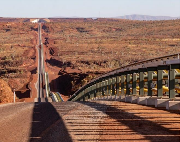
Overland Conveyor System
