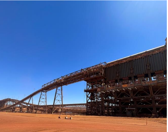
Ore Handling Plant 3
