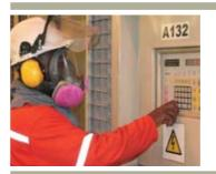
Programmable logic controllers help operators maintain optimum levels of alumina and terminate anode effects in cells at the Mozal aluminium smelter in Mozambiaue. This reduces emission of perfluorocarbon compounds, which are powerful greenhouse gases.
