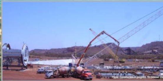
SOB Shuttle Train Car Dumper - Dumps ore from satellite ore bodies for blending and processing at the Newman Hub. Car dumper cell assembly completed in October 2008 (SOB = satellite ore body)
