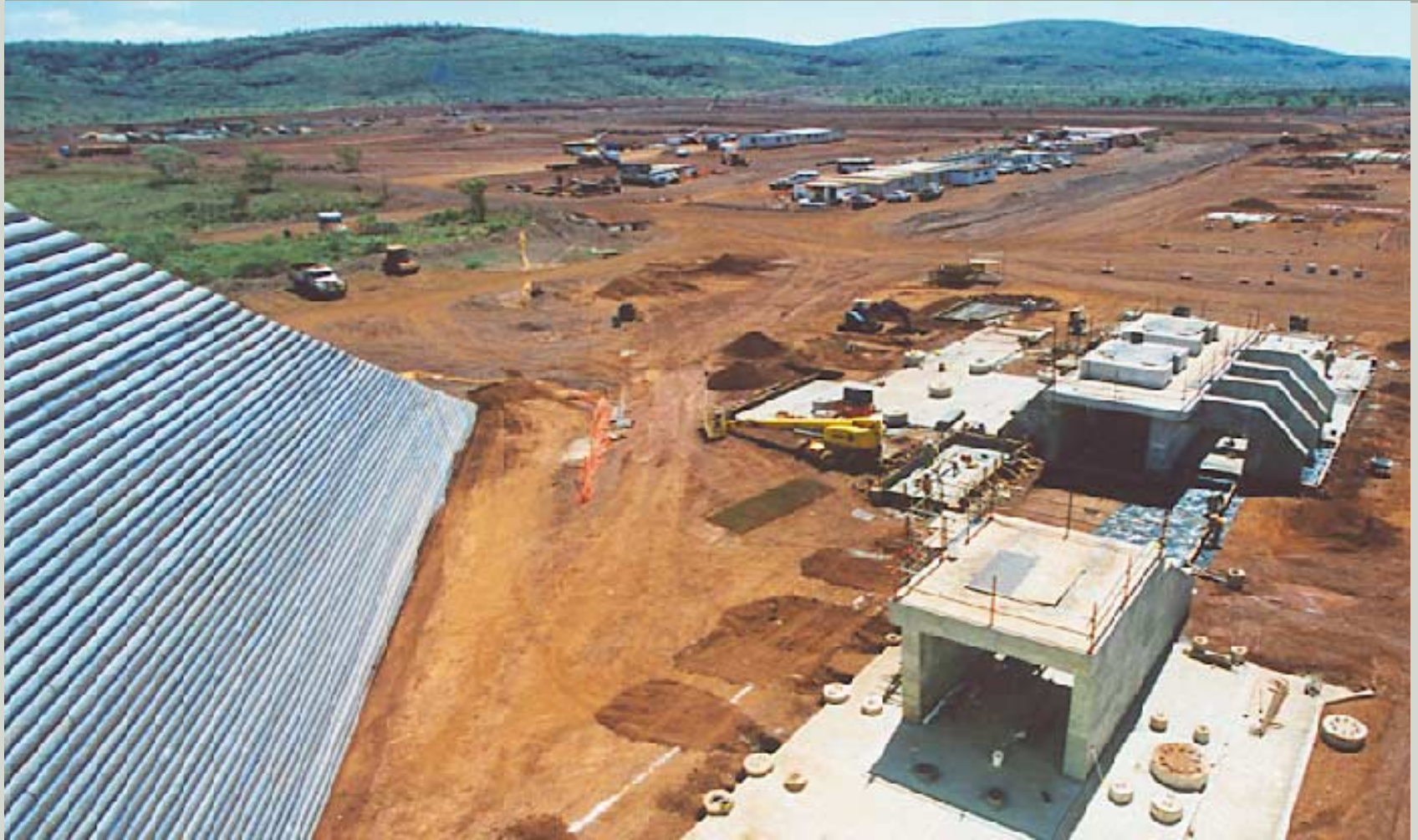
Picture: Foundations for Area C crusher
