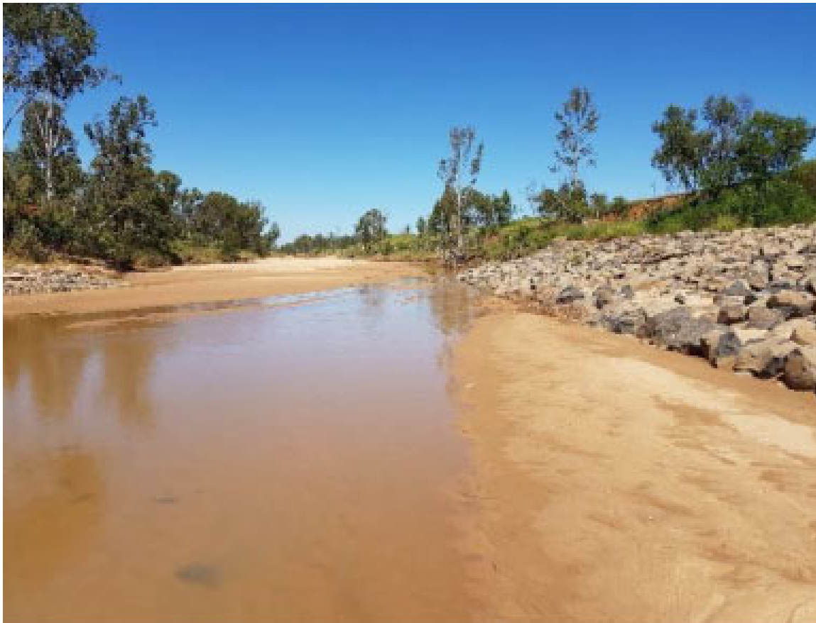
Plate 2 Armouring of river bank
