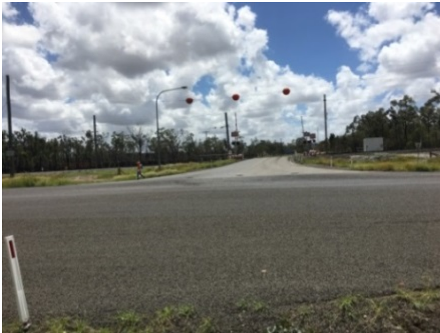
Plate 2 Dysart-Moranbah Road / Saraji Mine Entrance intersection
