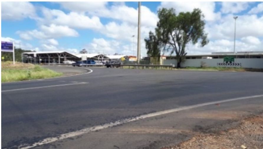
Plate 3 Dysart-Moranbah Road / Peak Downs Mine Road / Peak Downs Mine Entrance intersection
