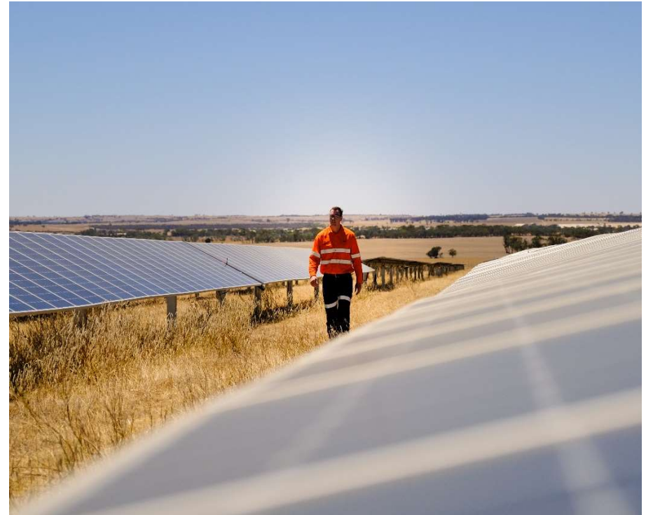
Merredin Solar Farm, Western Australia
