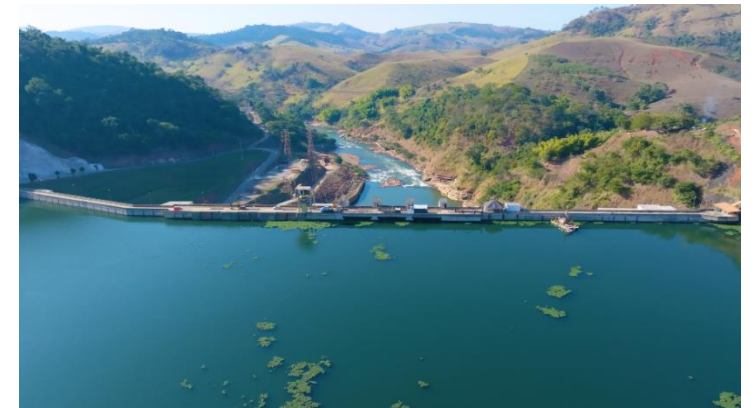
Candonga hydroelectric dam on the Doce River
