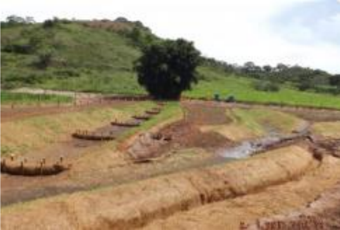
Reforming and stabilising drainage channels
