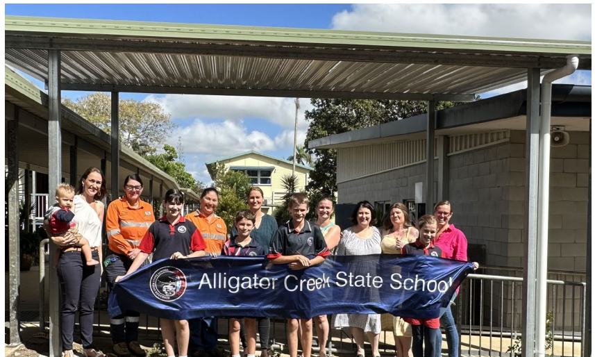
Alligator Creek State School's new undercover walkway was completed in 2023, with thanks to a grant from BMA. The structure provides protection from the sun and rain, keeping students and staff away from the impacts of weather.
