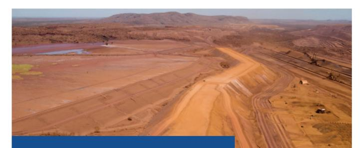
The Mt Whaleback TSF covers about 140 hectares, which is about 70 AFL fields. It's contained by a combination of natural ridgelines and man-made walls the tallest being about 26 metres high.
