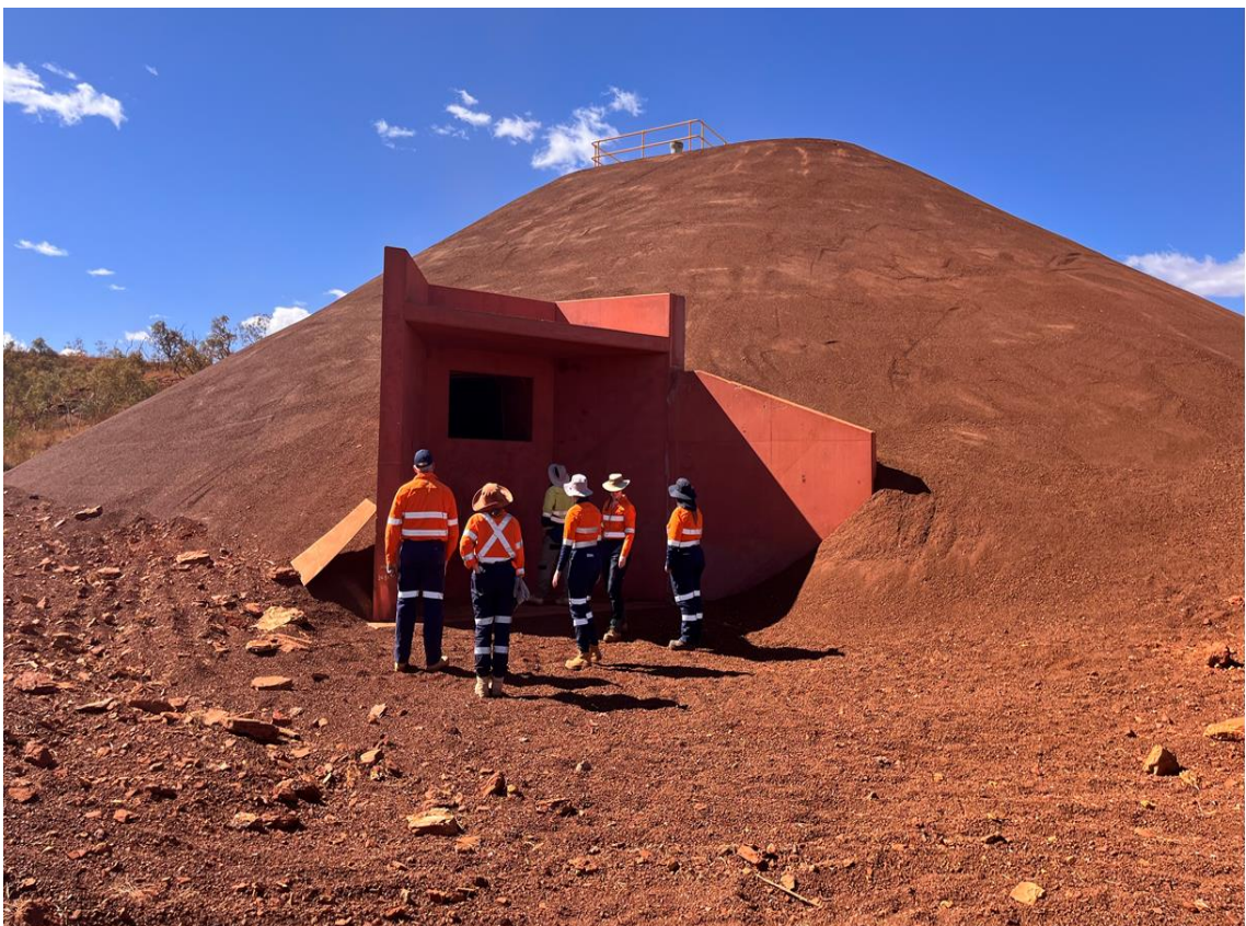
Figure 6-5 Completed Artificial Ghost Bat Roost (South Flank)
