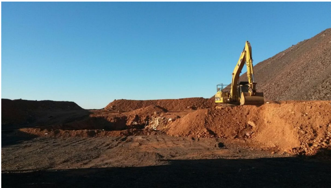
Plate 8.1 | Excavator and current waste dump face at the northern end of the landfill facility (May 2016)
