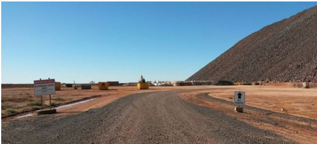
Plate 8.2 | Storage infrastructure (skip in foreground and various drums and containers in background) at landfill facility, looking south (May 2016)
