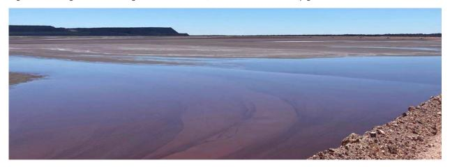
Figure 4.5 Tailings beach with active deposition, southern embankment spigot 13
