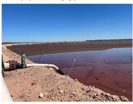
Figure 4.7 Freeboard capacity observation, southern embankment
