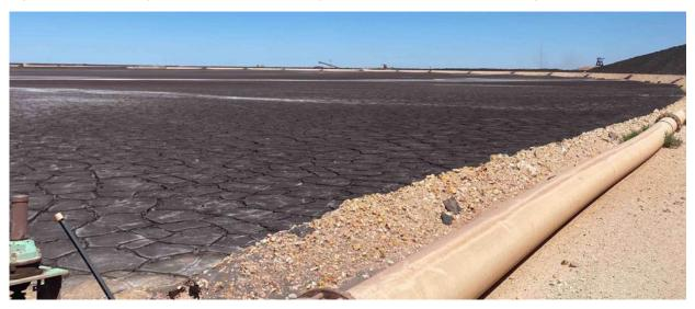
Figure 4.4 Tailings beach showing desiccation cracks, northern embankment spigot 14
