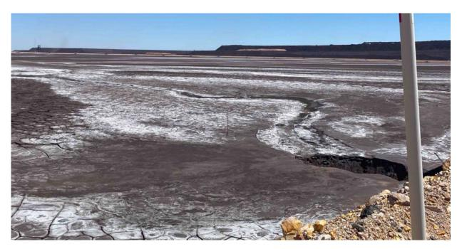
Figure 4.3 Consolidating beach development of tailings deposit, northern embankment spigot 25
