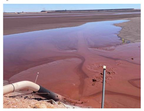
Figure 4.1 Discharge of tailings from Spigot 14 at the southern embankment, facing north
