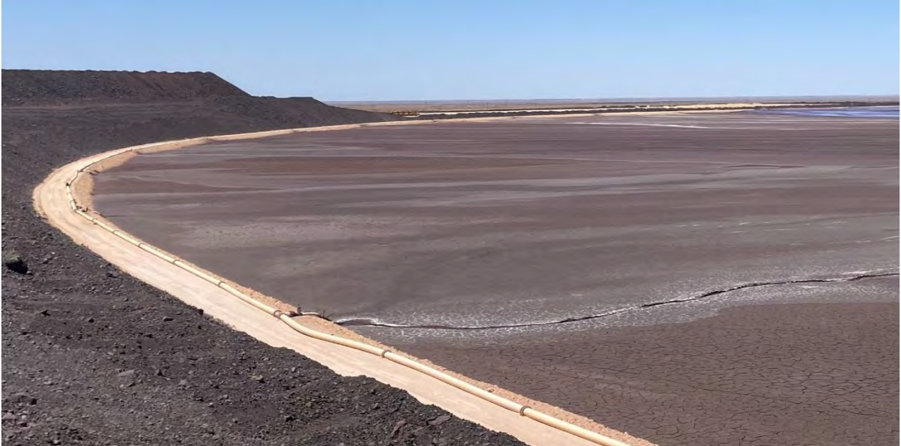
Figure 3.6 Freeboard capacity observation, northern embankment
