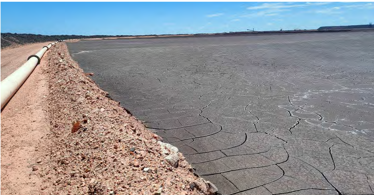
Figure 3.3 Discharge pipeline, southern embankment
