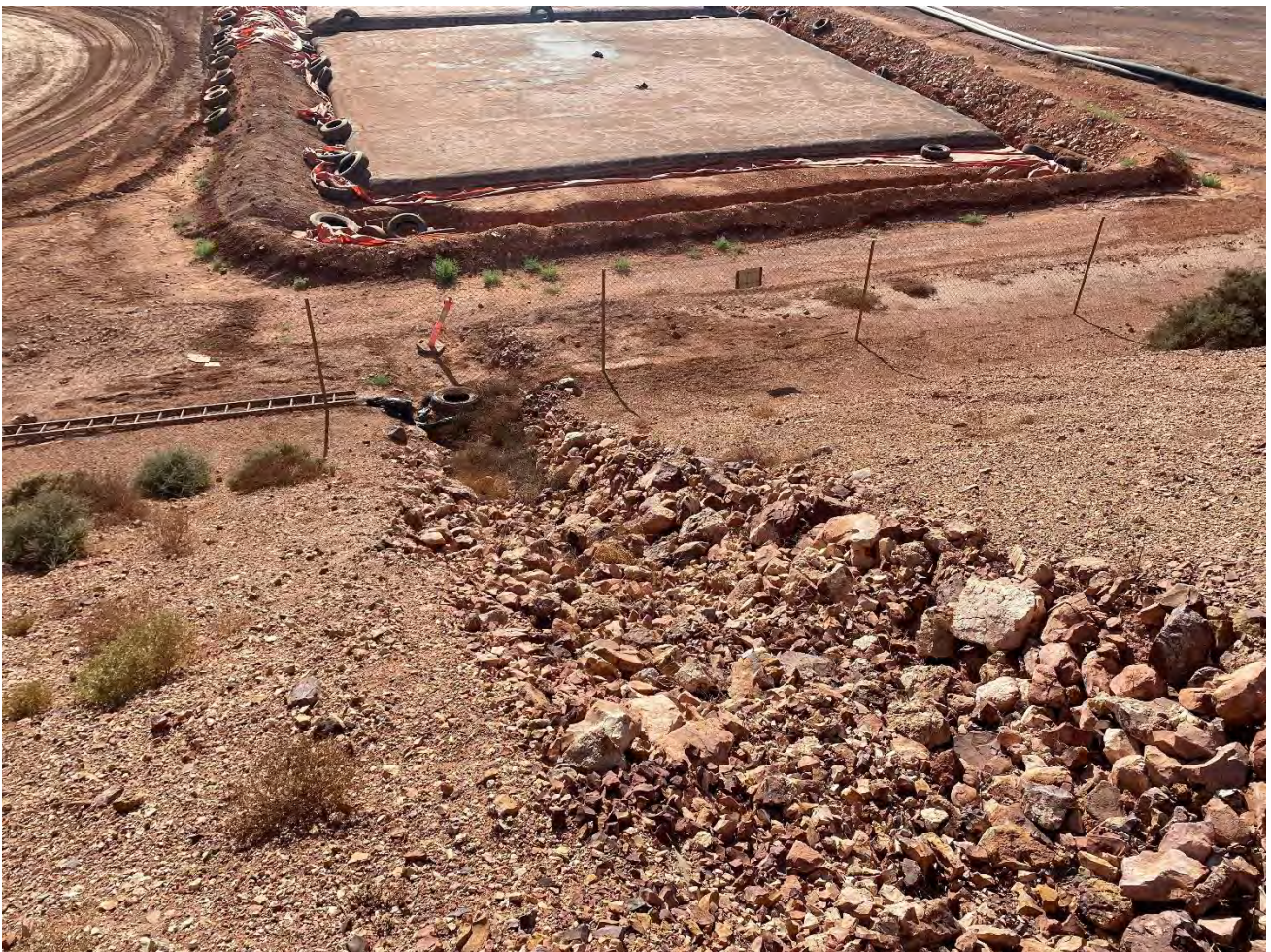
Figure 3.14 Raw Water dam spillway chute
