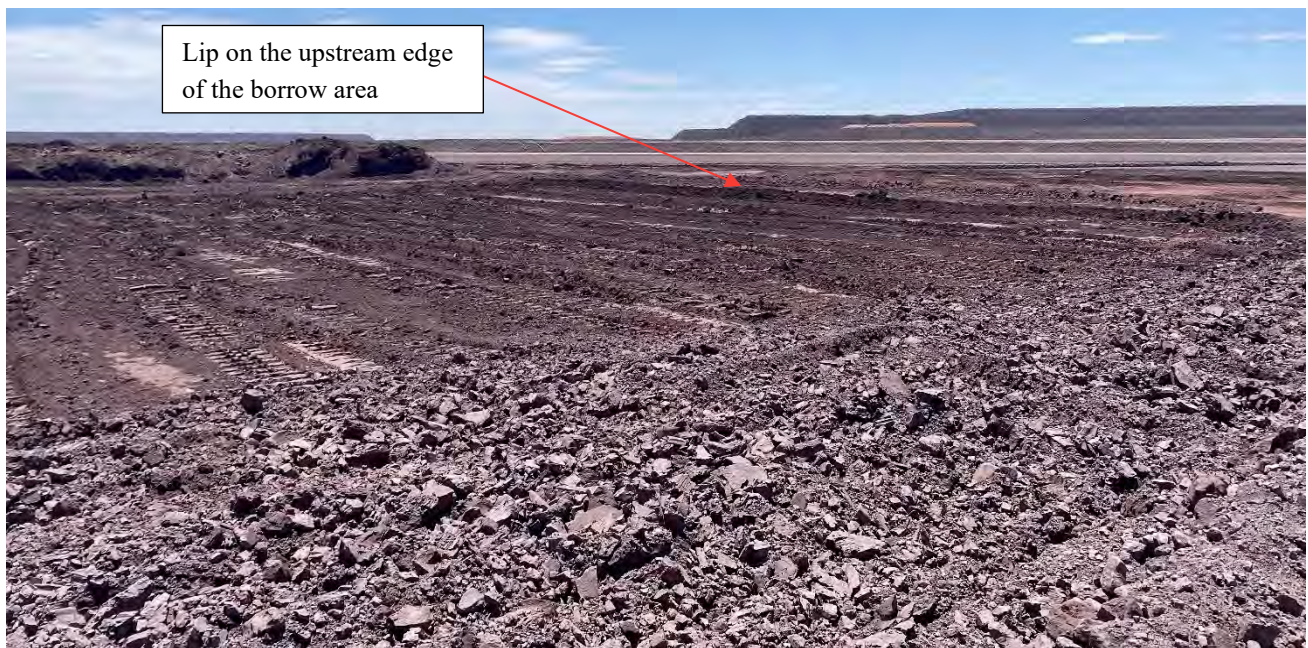
Figure 3.5 Tailings near to the southern embankment being tilled and piled up
