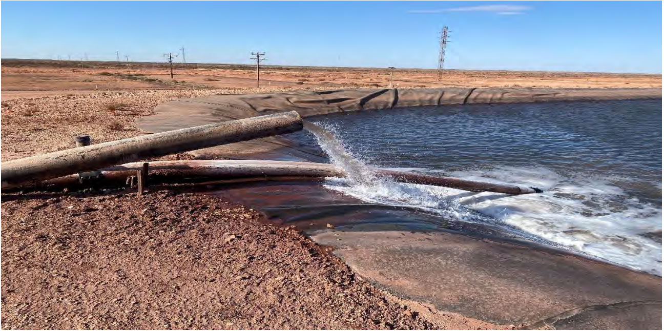
Figure 3.15 Discharge of water from the TSF into the Raw Water Dam
