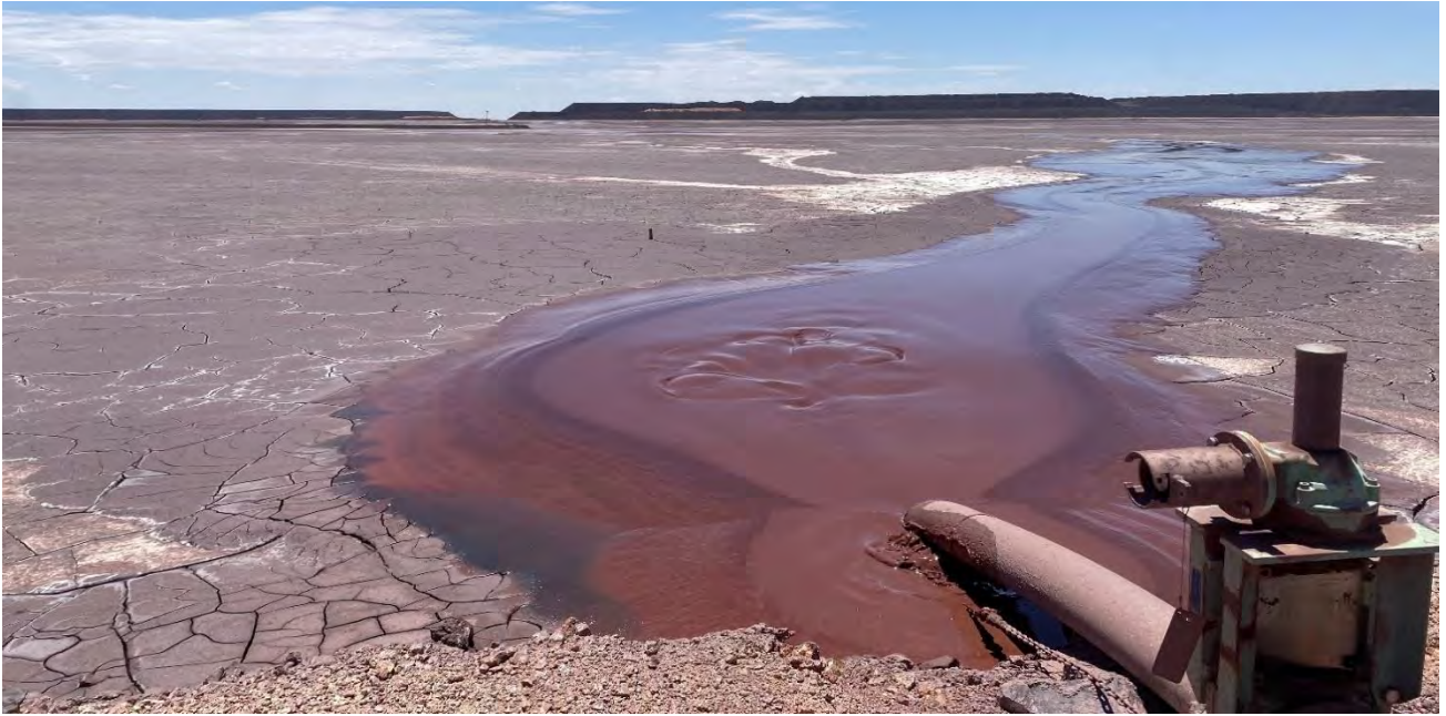
Figure 3.2 Tailings beach with active deposition, southern embankment spigot 15
