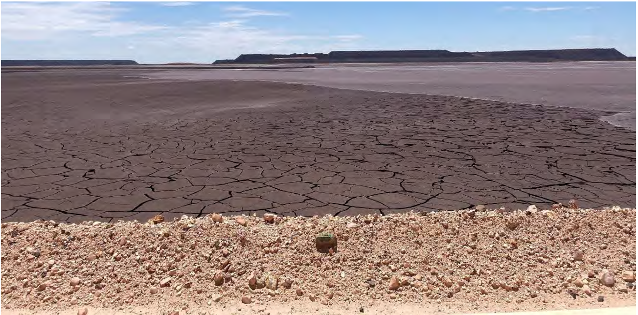
Figure 3.4 Tailings beach showing desiccation cracks, southern embankment
