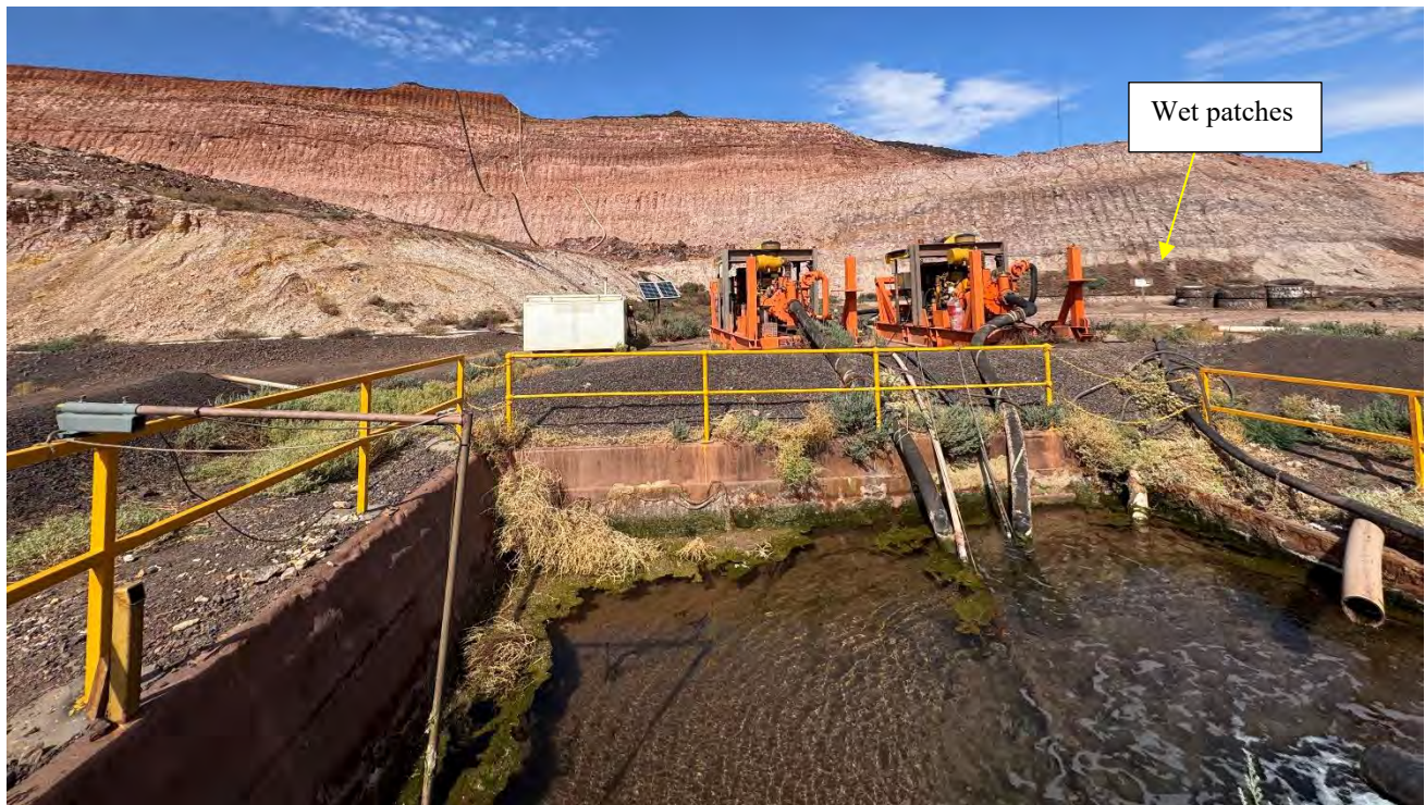
Figure 3.12 Damp spots on the face of the open pit, near the seepage collection sump
