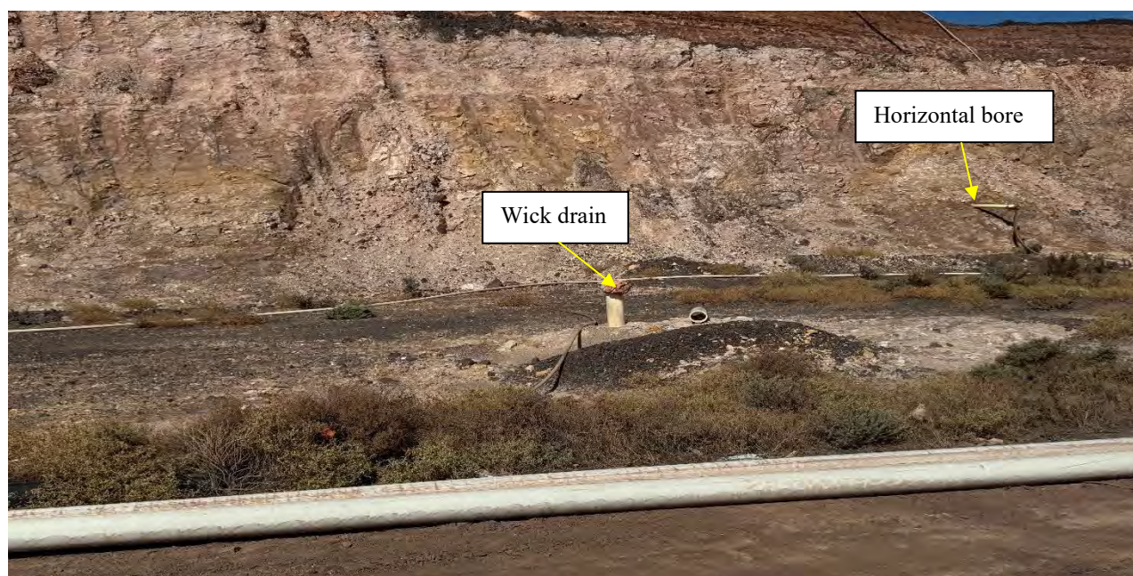
Figure 3.11 Example of a horizontal bore at the first bench of the open pit
