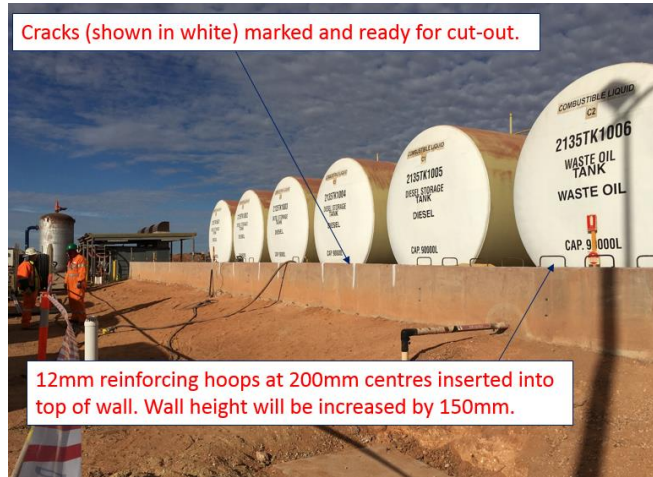
Figure 2.1-2: Upgrade and repairs to the mine end fuel bay.
