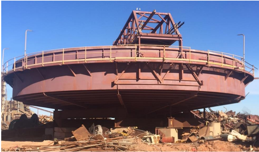
Figure 4.4-1: Legacy scrap steel stockpile (redundant tank) prior to removal.
