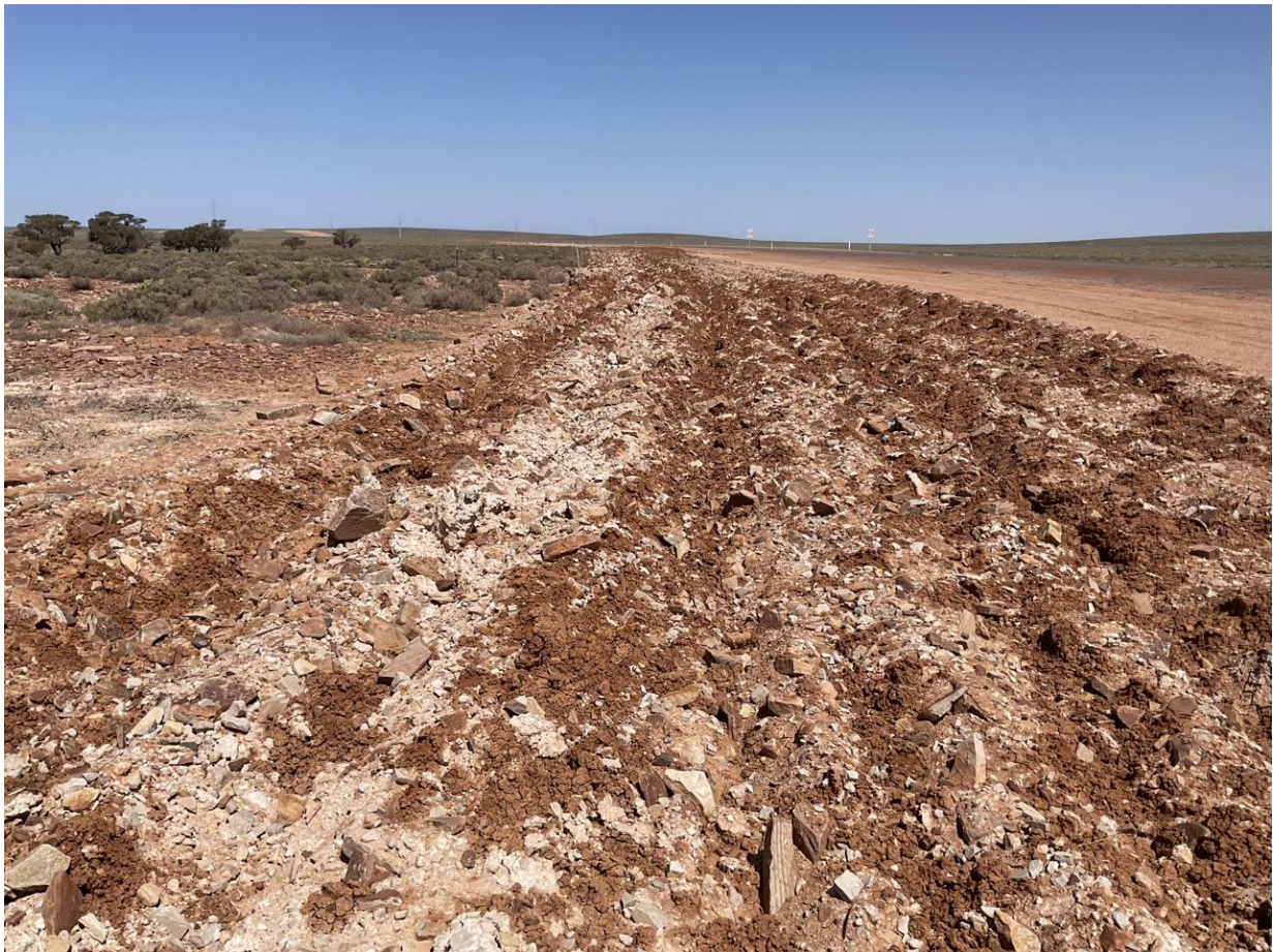
Plate 4.1: Deep ripped and hand direct-seeded section of WAR for proposed LFA
