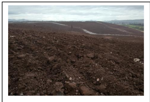
Natural rock in drainage lines to minimise erosion risk
