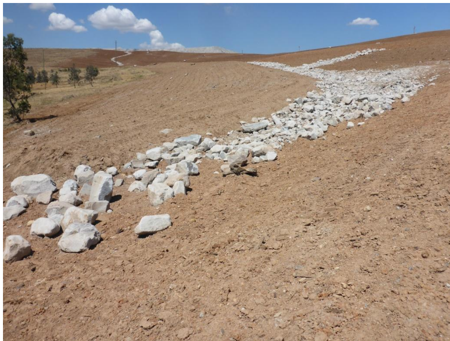
Plate 5: Example of Geofluv landform design implemented on site within the woodland rehabilitation. This area may require re-seeding, if germination is poor following decent rain.
