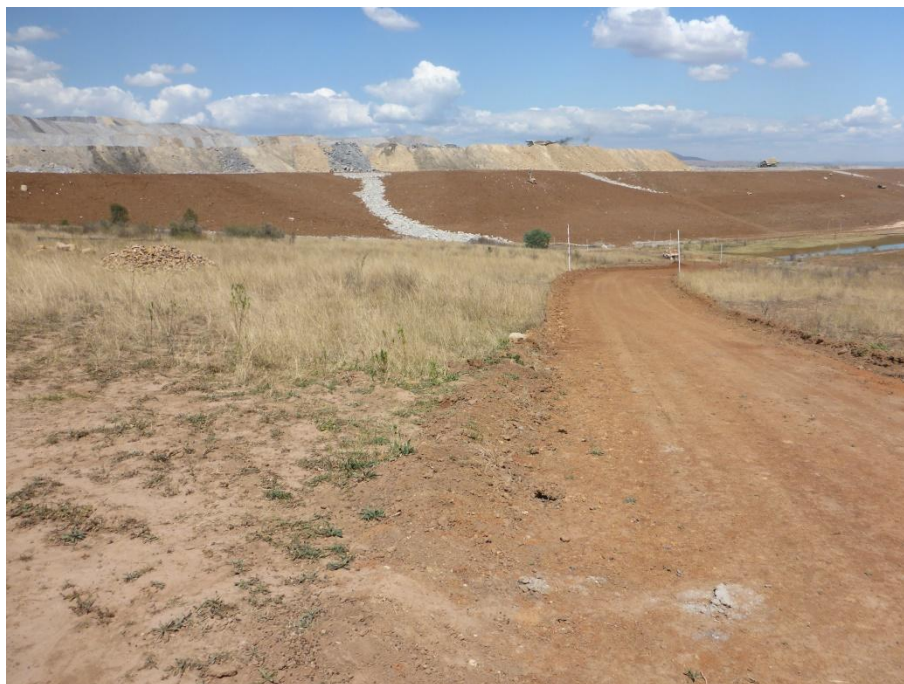
Plate 6: Example of Geofluv land form design implemented in the woodland rehabilitation. Also note the final dumping of overburden to design specifications to minimise dozer push on final landform. Evidence of the training and surveying/pegging procedure in action.
