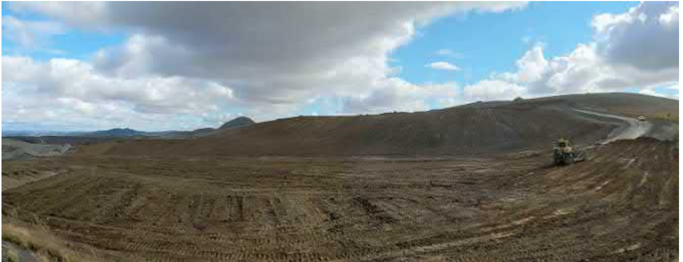
Figure 6: Topsoil spreading at Drayton Void emplacement
