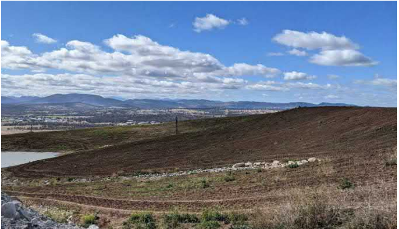
Figure 9 VD4 following maintenance work looking east
