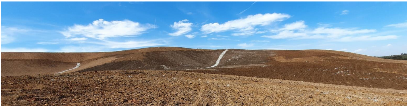
Figure 6: Rehabilitation at Saddlers Central emplacement using natural landform design
