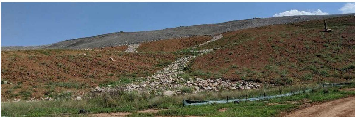
**Figure 7: Rehabilitation at VD5 emplacement using natural landform design**
