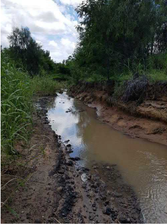
Figure 2-2: Spillway Channel Downstream of Dudley's Dam to Become Redundant
