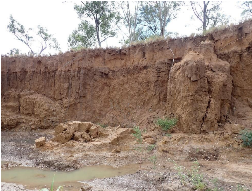
Figure 4-7 Bank collapse at site HC02 noted during the late-wet survey.
