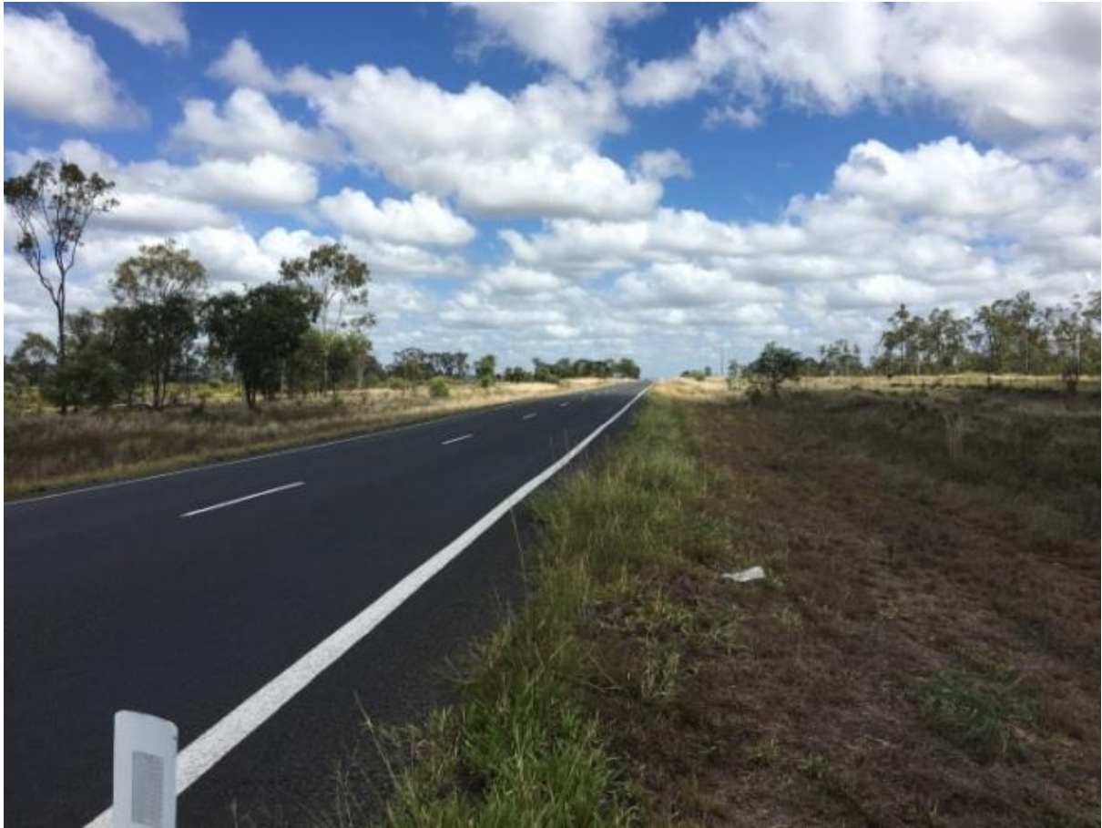
Plate 7 Road corridor at the proposed location of Intersection A (Saraji Road / the Project Site Entrance intersection)
