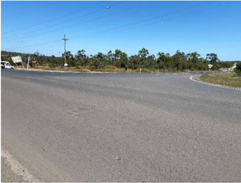
Plate 3 Saraji Road / Peak Downs Mine Road / Peak Downs Mine Entrance intersection
