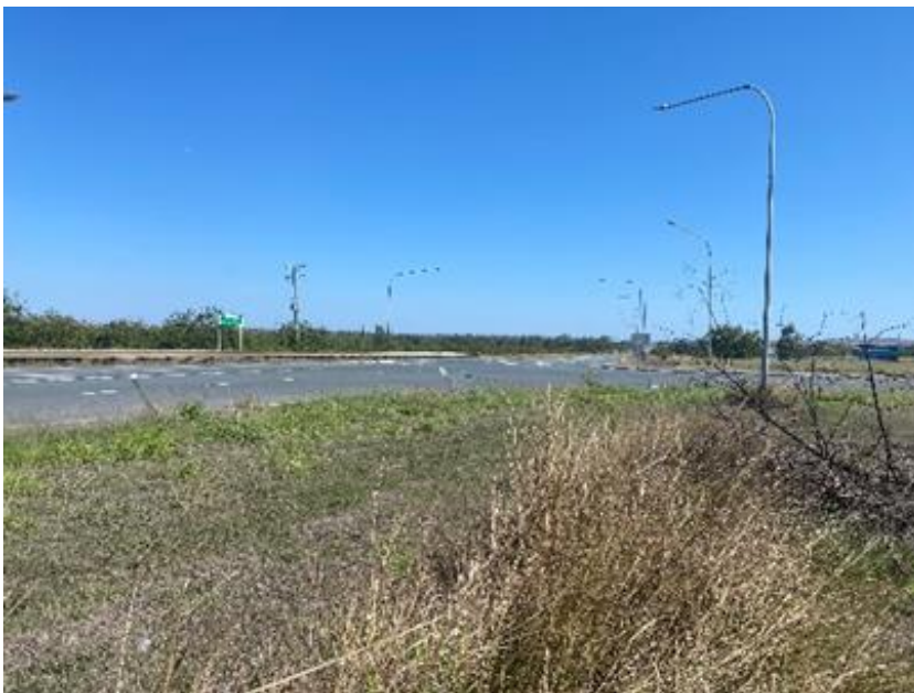
Plate 5 Peak Downs Highway / Moranbah Access Road intersection
