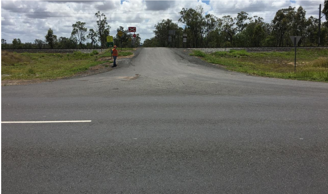
Plate 6 Intersection 1 (Saraji Road / Lake Vermont Road intersection)
