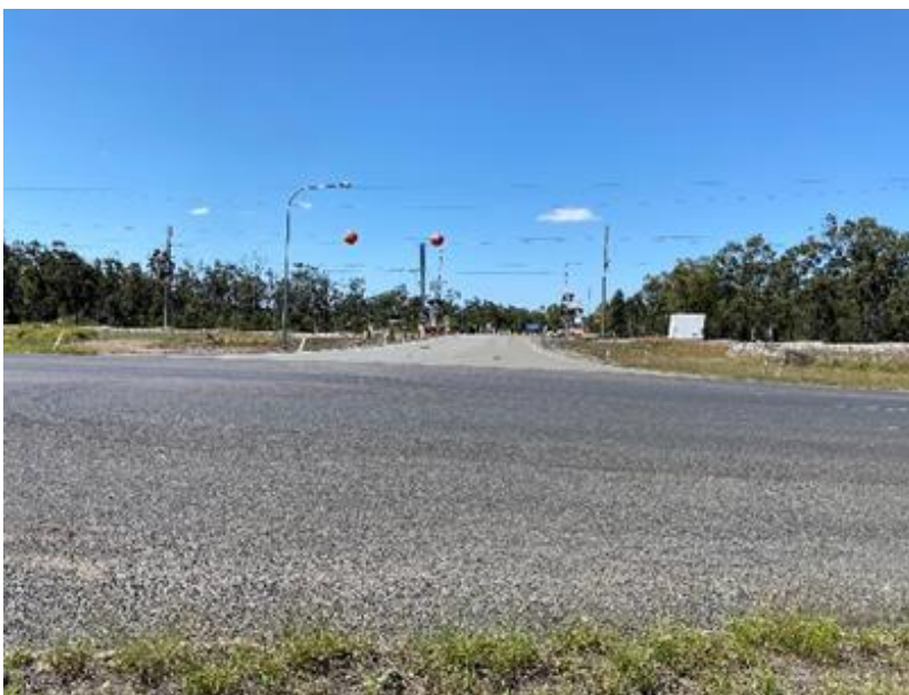
Plate 2 Saraji Road / Saraji Mine Entrance intersection
