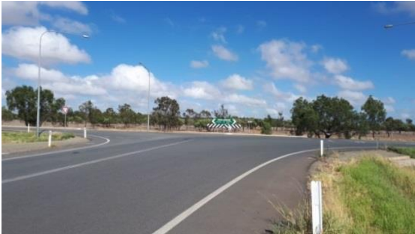
Plate 4 Peak Downs Highway / Peak Downs Mine Road intersection
