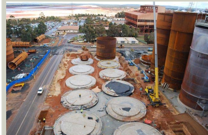
Precipitation Tanks & Pre-assembly
