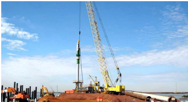
First RGP5 wharf pile being driven in
