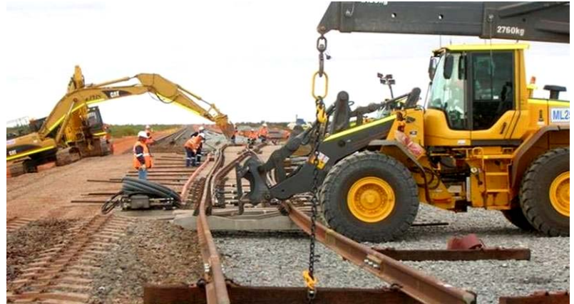
Turnout installation at Bing South
