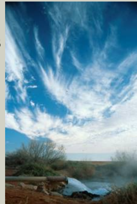
After bore capping
