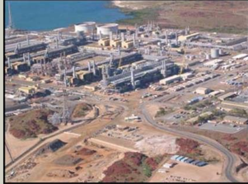
Onshore Gas Plant pre-Train 5
