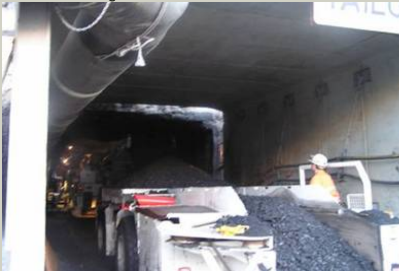
Producing coal at Broadmeadow June 2004
