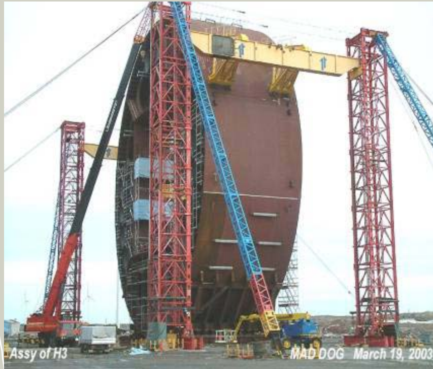
Spar Construction
