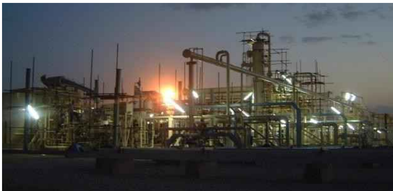
SUNRISE OVER THE ZAMZAMA GAS PLANT DURING CONSTRUCTION
