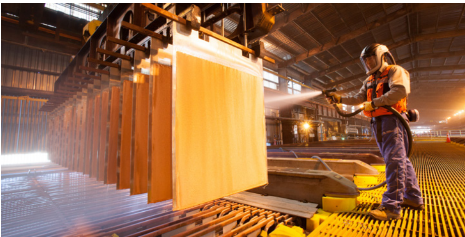
Exposure control at Escondida copper cathode plant in Chile.
