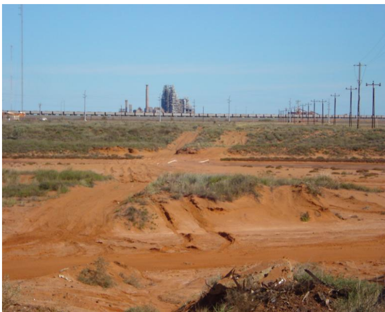
Plate 17: Decommissioned Boodarie Hot Briquette Iron Plant as Seen from Pinnacle Road Wedgefield.
