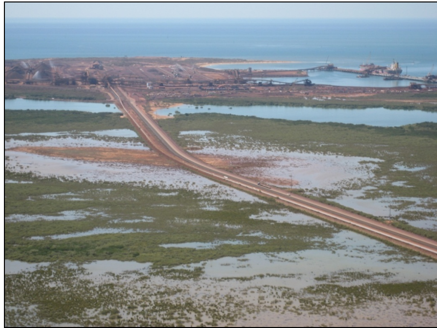
Zone 1: Aerial photograph showing existing road and causeway to Finucane Island (located in background). Existing BHP Billiton Iron Ore operations on Finucane Island can be seen. Mangroves and tidal flats are located either side of the existing road. The proposed conveyor system is to be located to the west of the existing road.
