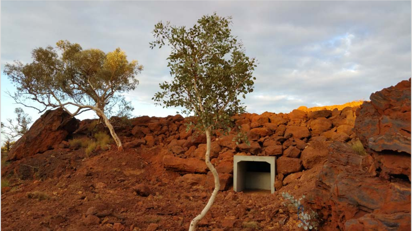
Completed artificial ghost bat roost constructed in the vicinity of Mining Area C
