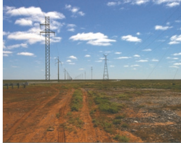
Plate 2.16 The existing 275 kV and 132 kV transmission lines
