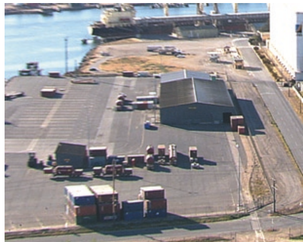
Plate 2.17 Aerial view of the existing BHP Billiton Port Adelaide loading and unloading facility at Berth 25
