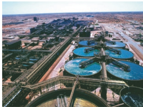
Plate 2.8 Countercurrent decantation circuit
