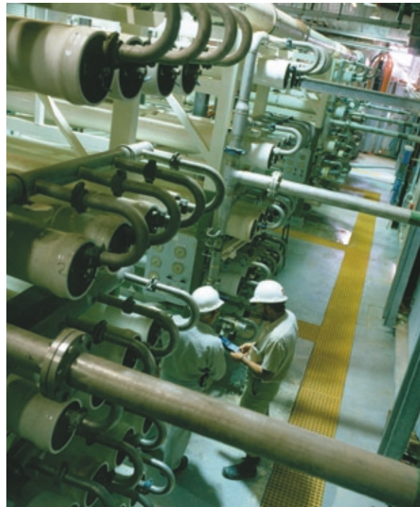
Plate 2.15 The on-site desalination plant produces about 14 ML/d of desalinated water
