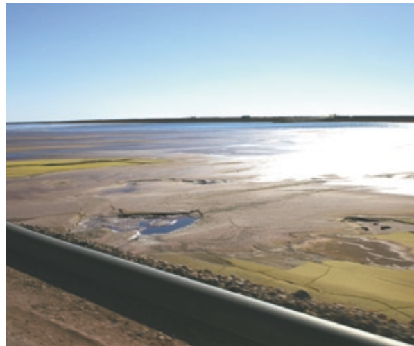
Plate 2.12 The existing tailings storage facility cell 4
