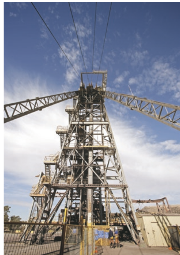
Plate 2.5 Whenan Shaft is one of the two operational shafts at Olympic Dam
