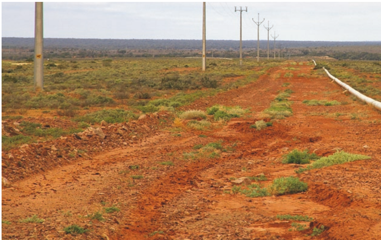
Plate 20.5 Existing SA Water pipeline and transmission line near Woomera
