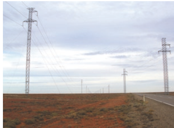
Plate 20.4 Transmission line crossing the main road between Roxby Downs and Woomera
