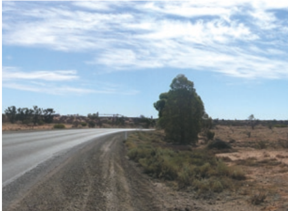
Plate 20.1 Existing mine infrastructure visible on the skyline at Olympic Dam
