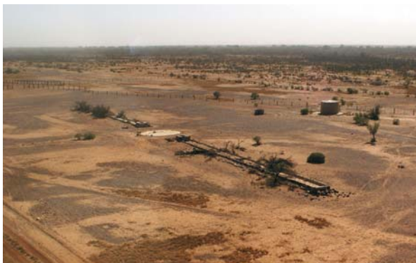
Plate 18.12 Junction Well trough
