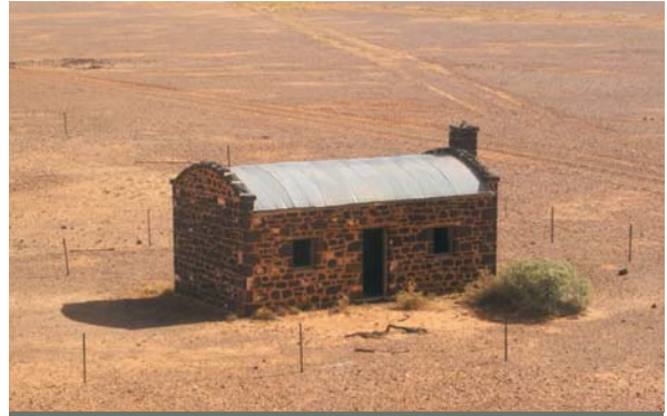
Plate 18.13 Junction Well hut
