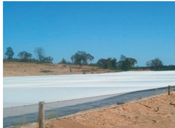
Plate 15.29a Example of netting to exclude birds from a mine dewatering pond
