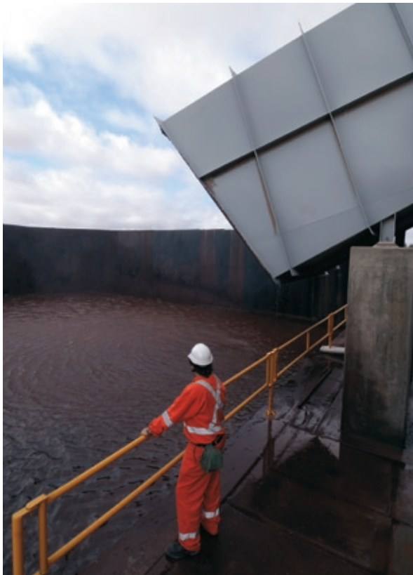
Plate 13.5 Saline aerosols capture infrastructure
