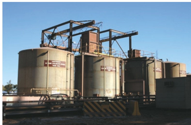
Plate 13.10 Reagents storage area
