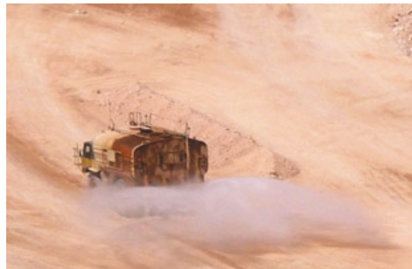
Watering a haul road to reduce dust generation
