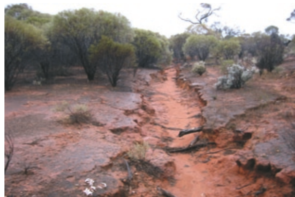
Plate 11.7 Erosion due to concentration of stormwater flow through culverts
