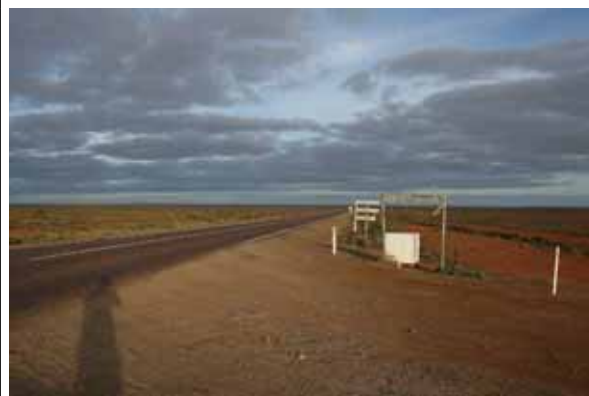
Photograph 12 Typical minor priority intersection without right-turn reserve and merging / diverging lanes
