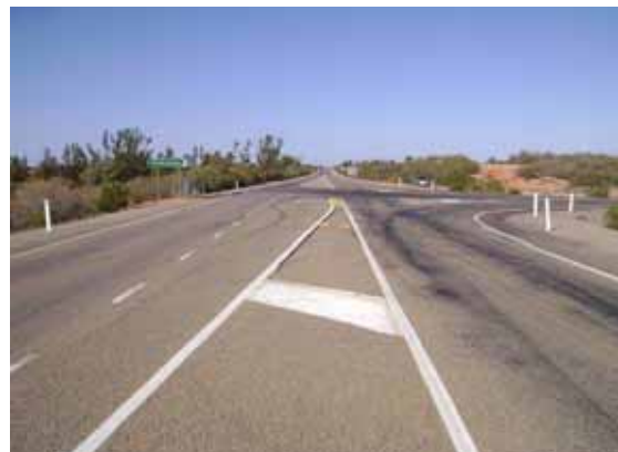
Photograph 11 Typical priority intersection with right-turn reserve and merging / diverging lanes
