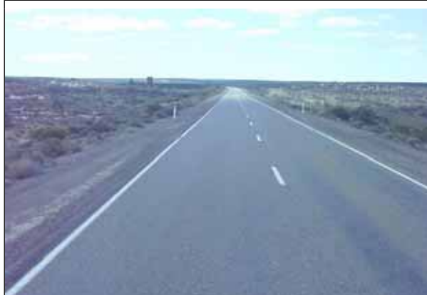
Photograph 10 Olympic Way (Pimba to Olympic Dam)
