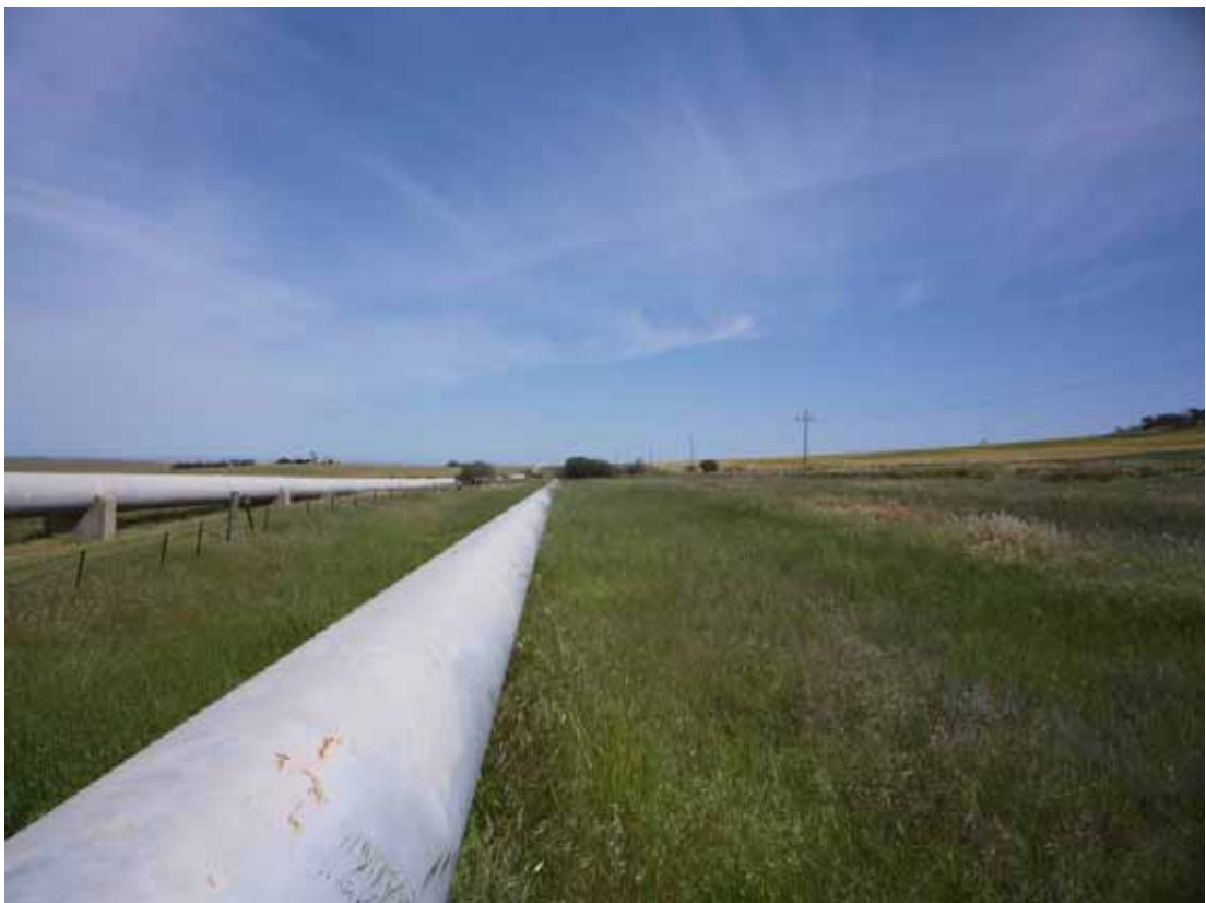
PHOTOGRAPH 3.2 General photo of the general location for the new Hughes Gap PS
