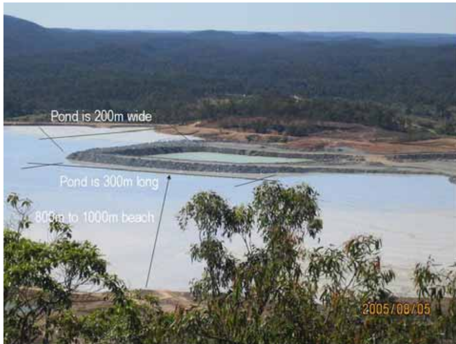
Figure 6.5 Rock Decant Control Wall (Photo courtesy Mt Rawdon Gold mine)
