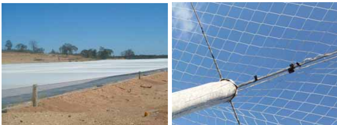
Figure 6.6 Bird netting (NetPro) over pond (photos courtesy of AusLive Fish Farm Calliope, Queensland)
