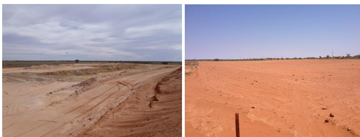
Figure 1.1-11: Borrow pit rehabilitation works (before left, after right)
