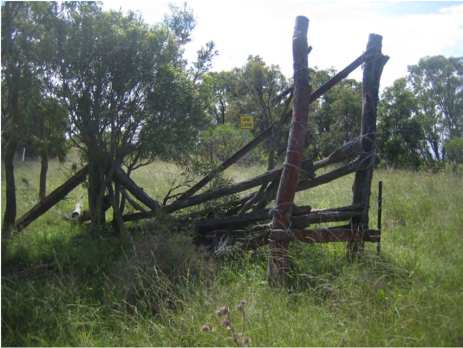
Plate 1: Remains of loading ramp
