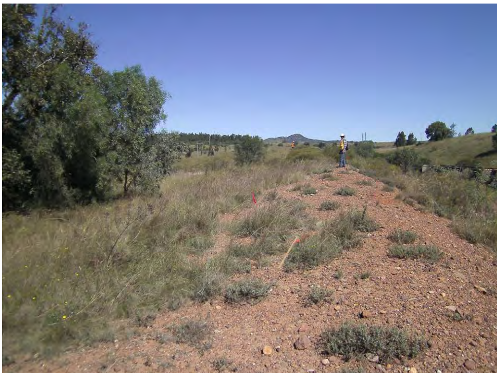
Plate 2: AS2 view south west showing site on embankment
