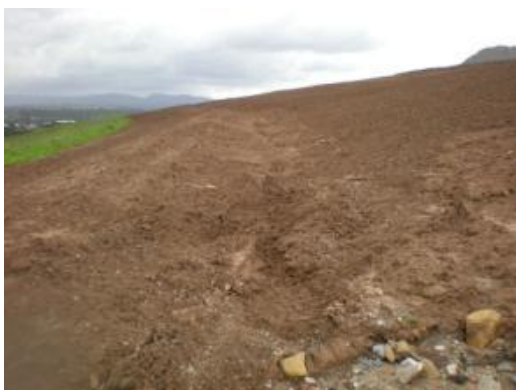
Plate 5: Spoil emplacement VD1 contoured and top-soiled for revegetation.
