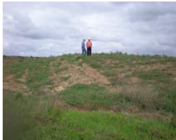
Plate 4: Windmill topsoil stockpiles showing dispersive soils and weed infestation.
